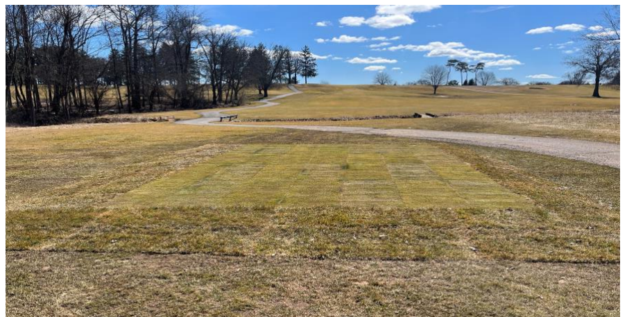
16 th Green/White Tee Rebuilt to double the size
